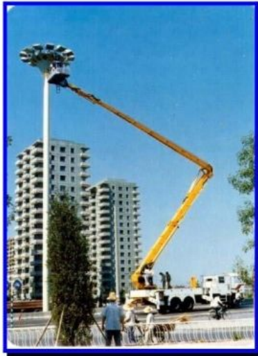
Street Lighting maintenance
